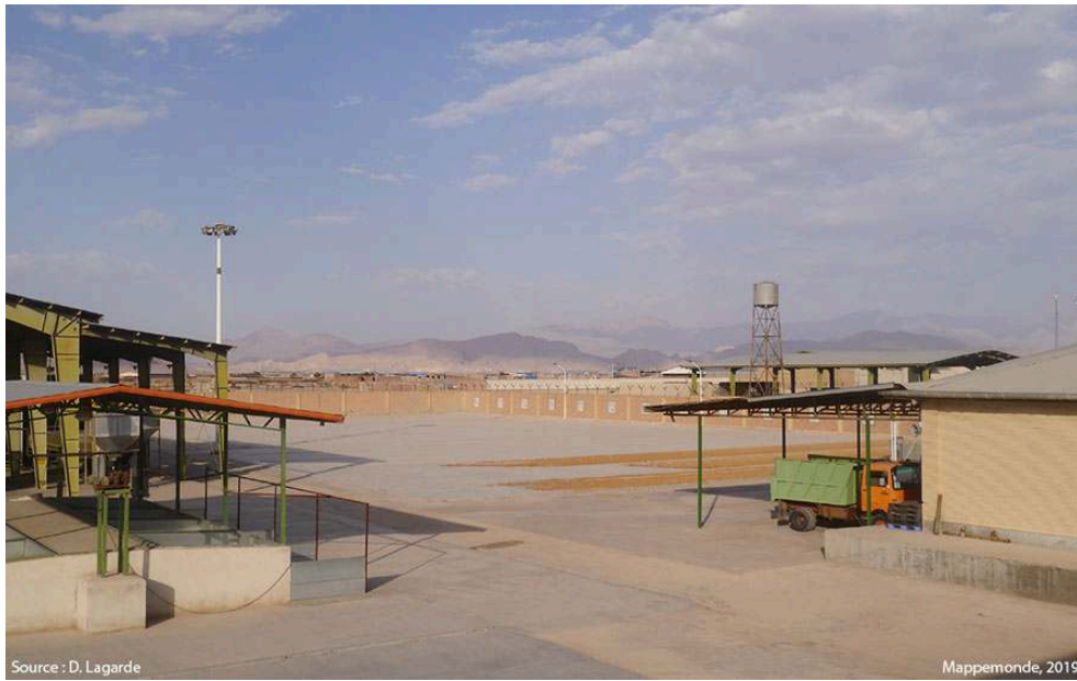
Figure 9. Pistachio packing plant in the city of Kerman (Iran)
