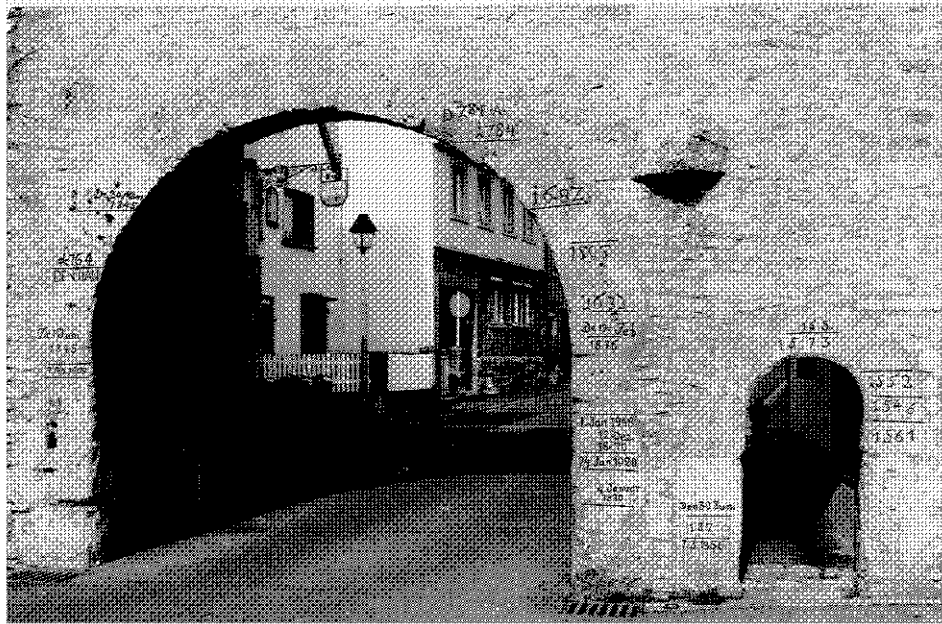
Figure 2. Marks of water levels on the Main Gate in Eibelstadt, Germany (Photo: R. Glaser).
